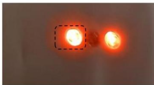
Picture11. Battery out
